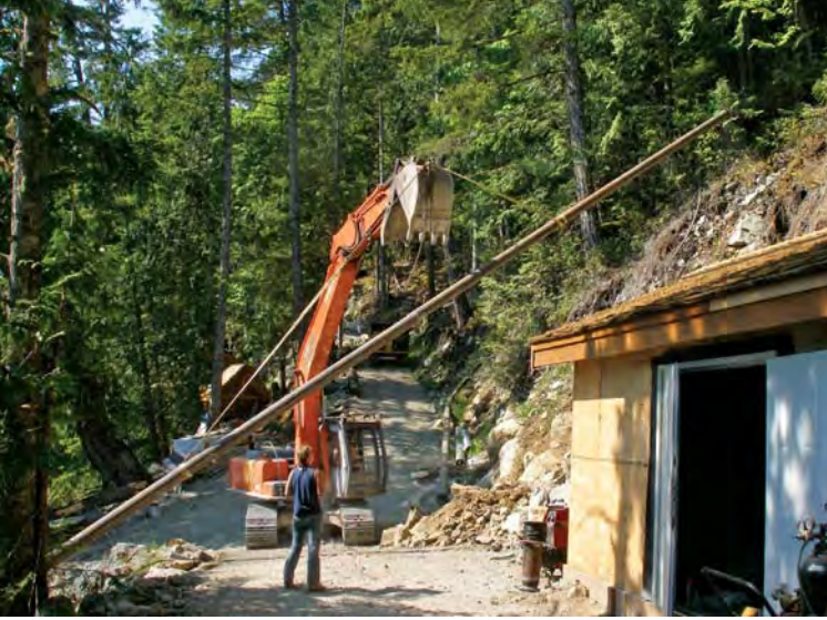
An excavator lifting a 3,000-pound section of 8-inch steel onto a steep slope. The pipe was then pulled 500 feet up the hill using the excavator and a long steel cable through a pulley.
