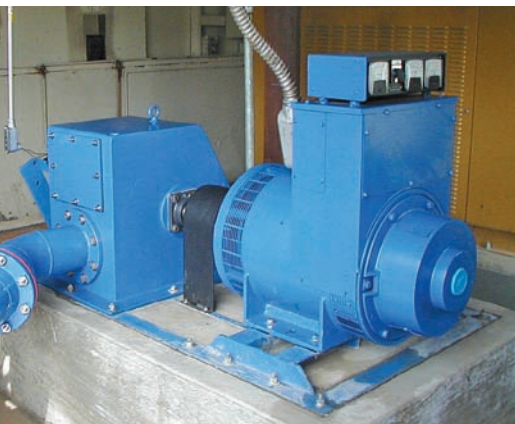
One of the smaller turbines from Canyon Industries, this 16 KW Pelton unit powers 120 and 240 VAC loads directly without batteries or inverters.
