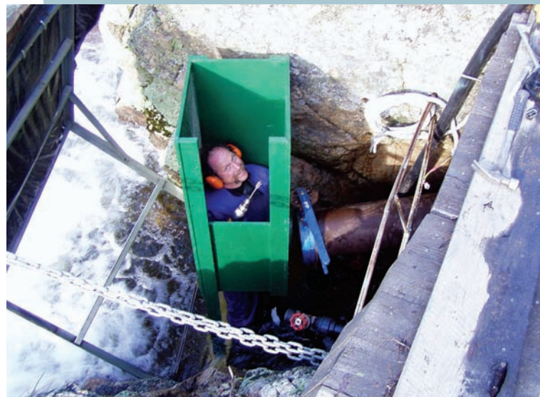
The author works on attaching the penstock to the stand box.
