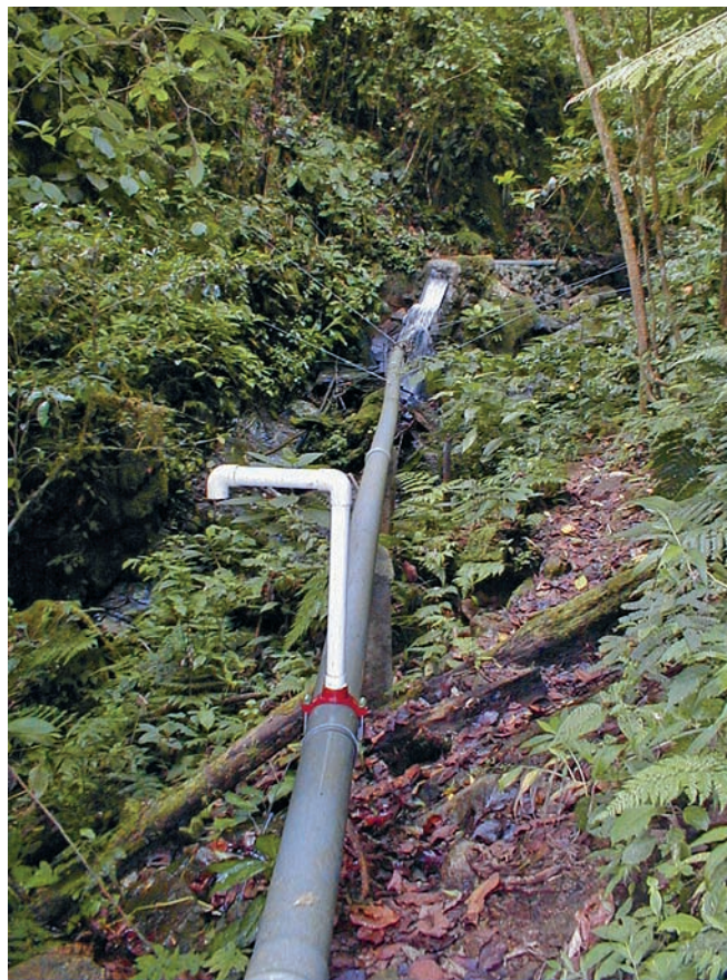
Intake and top section of penstock with standpipe vent.
