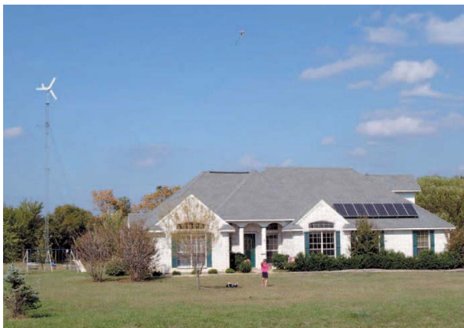
The Geislers' RE-powered home, AWP 3.6 wind generator, and recently added PV system.
