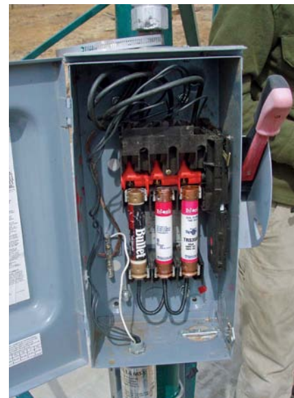
Dynamic braking uses the alternator's electromagnetism against itself by shorting all three wires together.
