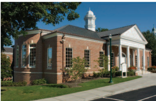
The Glenn Building is heated and cooled by an efficient geothermal system.
