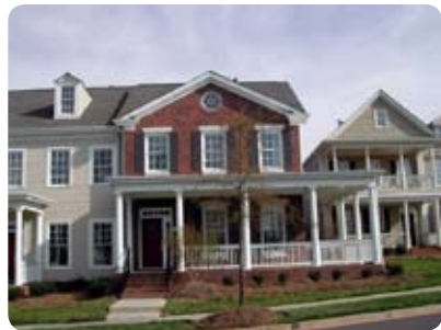
Mix of housing types in a new neighborhood
