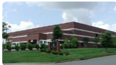
Industrial, warehouse, or distribution-type building
