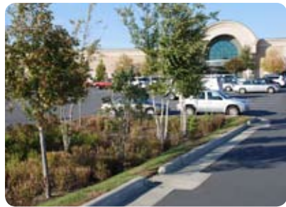
An example of a bio-retention area in a mall parking lot in Charlotte, NC. The curb cuts allow stormwater to enter the retention area.
