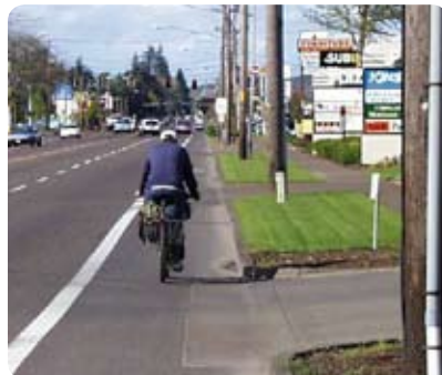
Bike lane added to a 5-lane commercial corridor through travel lane narrowing, which also contributes to increased safety for motorists and decreased speeding.
