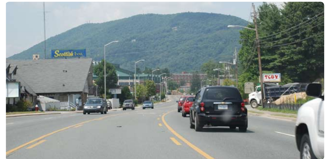
Existing conditions on US 321 between NC 105 and Rivers Street. Uncontrolled access, frequent driveways, and limited or low quality bicycle and bicycle facilities add to congestion and safety problems for all users along the roadway.
