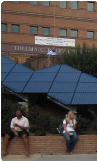
A recent installation of solar panels on the ASU campus
