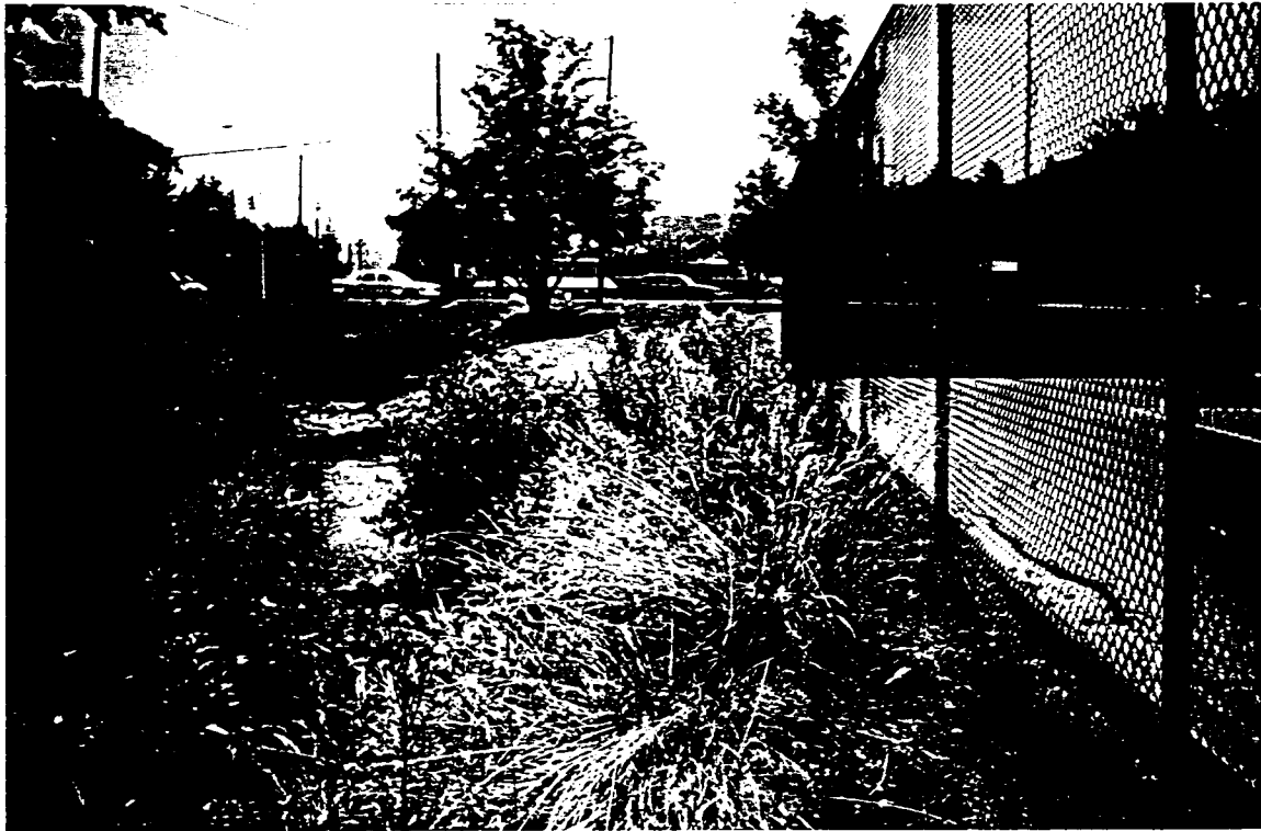
Photo 4. Looking downstream at arch culvert under Rivers Street at US 321. Note ASU tennis courts adjacent to Boone Creek channel.
