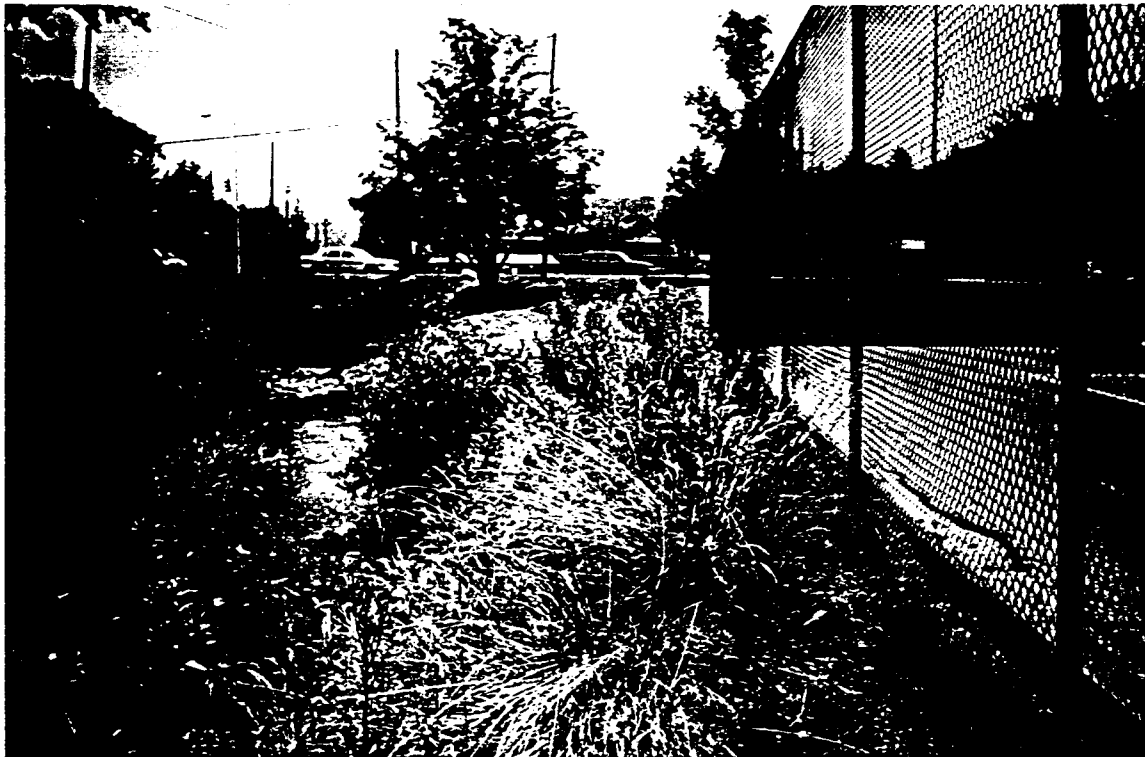
Photo 4. Looking downstream at arch culvert under Rivers Street at US 321. Note ASU tennis courts adjacent to Boone Creek channel.
